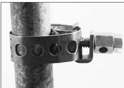
Step 12 - Insert Bolt Through Both Copper Holes & Tighten using a 7/16" Wrench
