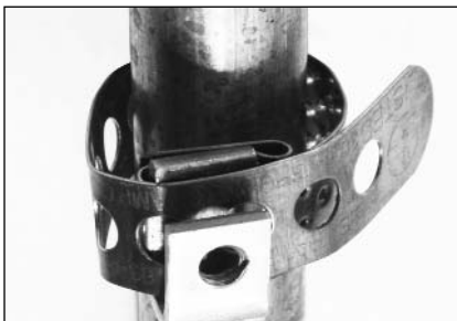
Step 11 - Wrap Strap Tight Around Pipe
